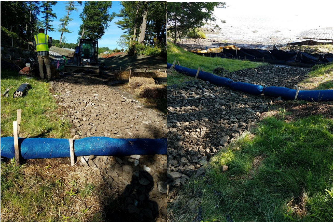
Figure 4. Restored lower slope, completed July 1, 2020. Remaining restoration was completed July 2, 2020.
